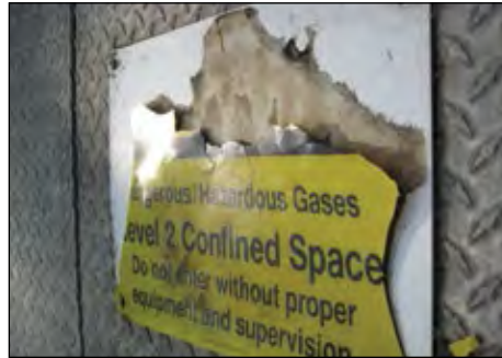
Delaminated Metal
